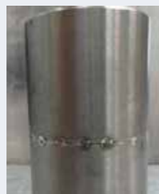
Pipe butt weld Ø 31,75 x 2 mm.
